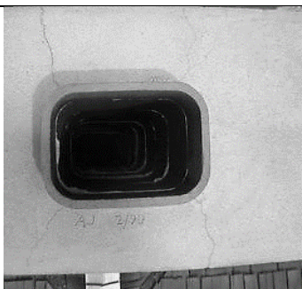
Clay Tile Liner Flue
