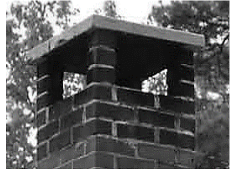
Concrete Cap Chimney Top
