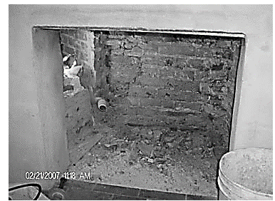
Badly Deteriorated Firebox
