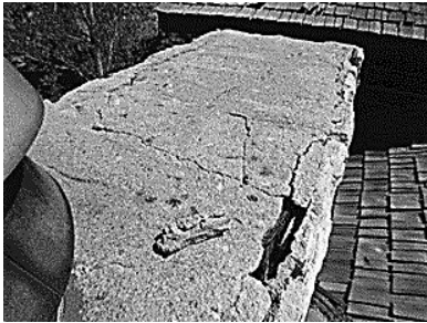
Damaged Chimney Cap
