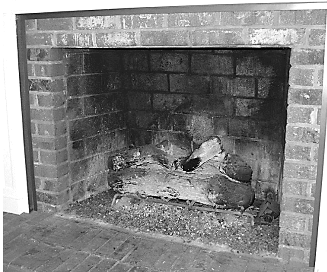
Masonry Woodburning Fireplace insert
